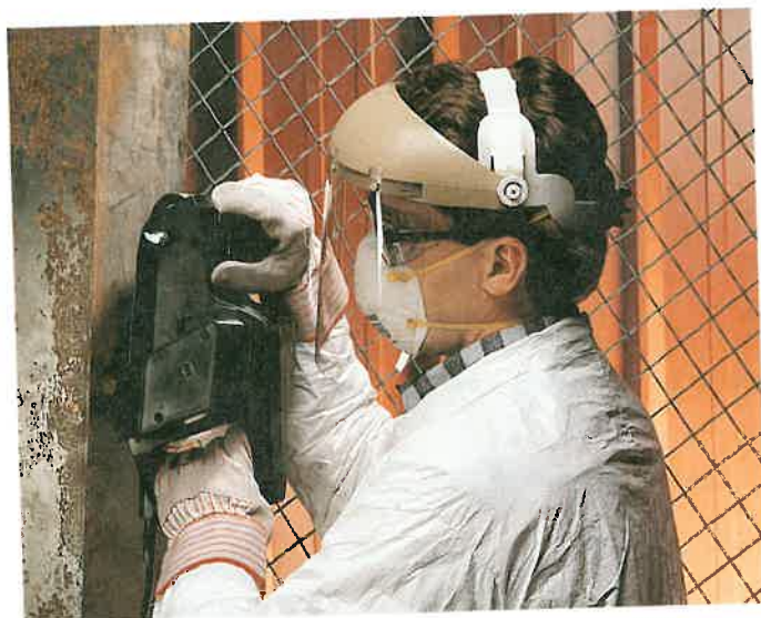
Figure 18-18. While sanding, it is advisable to wear a face shield and some form of respirator. (Lab Safety Supply Co., Inc.)
