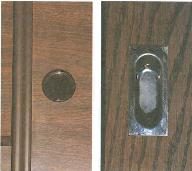
Figure 17-3. Flush mount pulls do not interfere with sliding doors.
